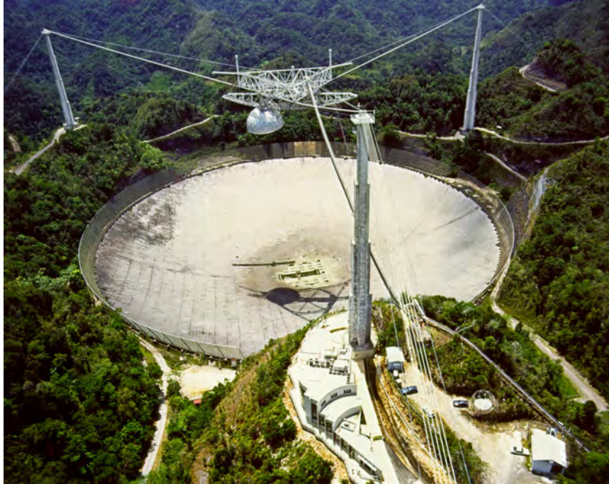
Fig. 5.16 The 305-m diameter radio telescope at Arecibo, Puerto Rico. Image credit: Wikipedia
