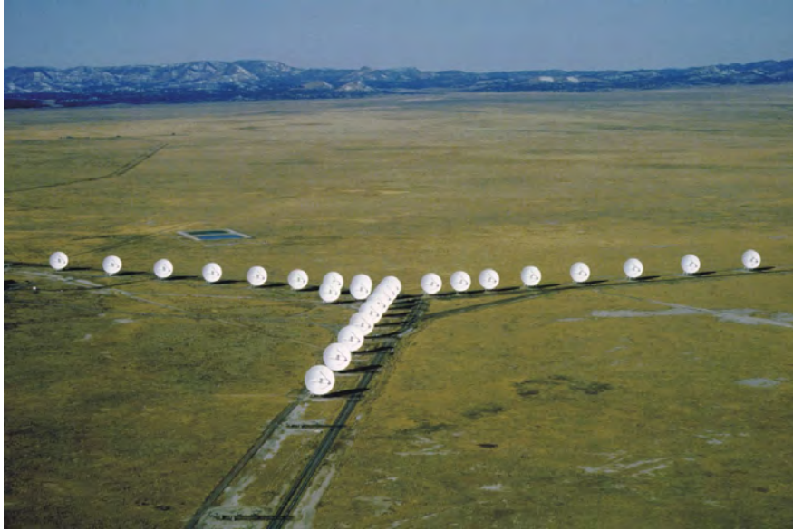
Fig. 5.8 The Very Large Array (VLA) in New Mexico. Each dish antenna is 25 m in diameter. The separation between the individual dishes can be changed to generate different desired beamsizes. Image credit: NRAO/AUI
