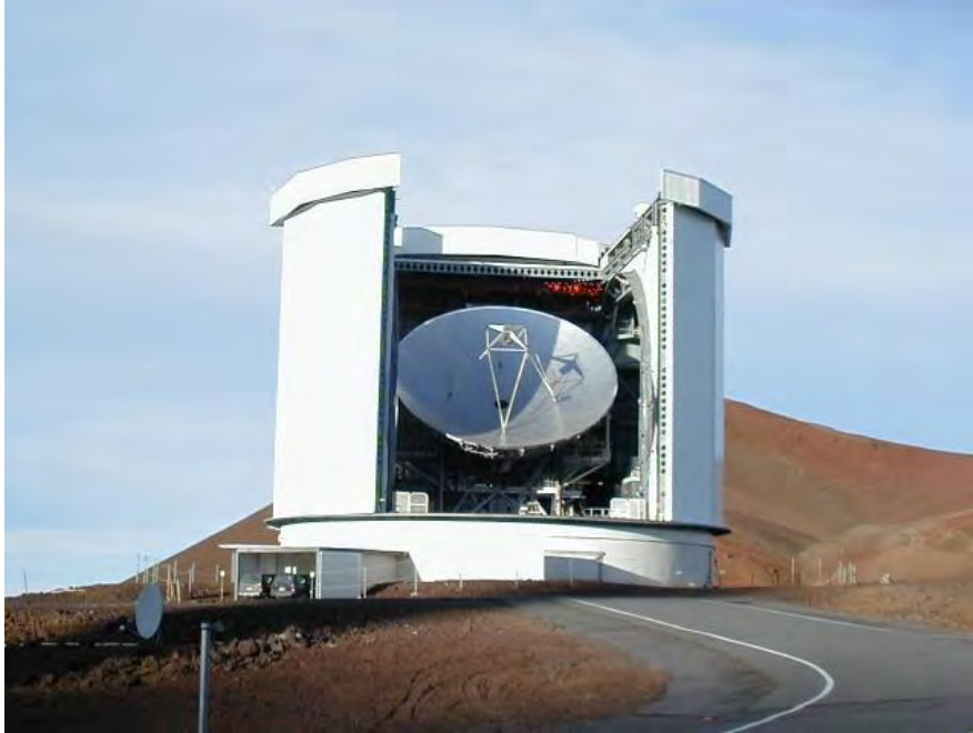
Fig. 6.12 The JCMT telescope on Mauna Kea, Hawaii. The telescope is usually protected from the wind by a Gore-Tex membrane which fills the opening of the dome. Image credit: UK Scientific & Technical Facilities Council
