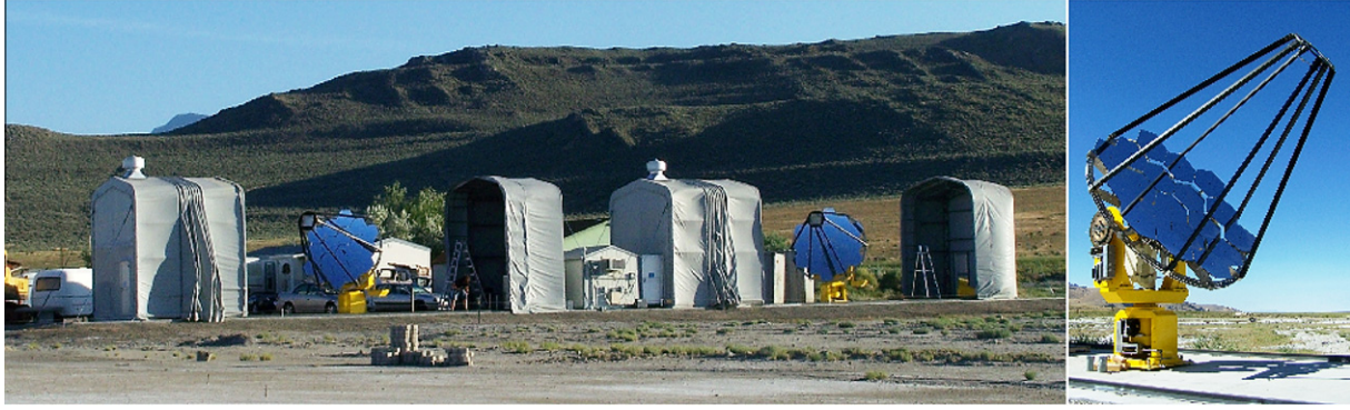
Fig. 10. The StarBase 3m telescopes are protected by buildings which can be rolled open for observation (left). The control room is located in a smaller building located between the two telescopes. Right: Close-up view of one telescope.
